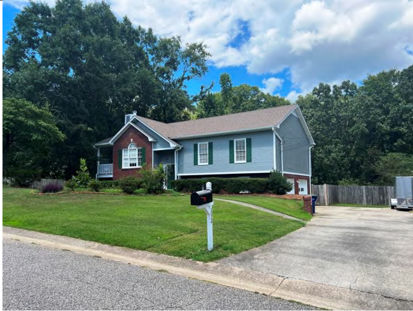
Photographer: Tyler Powell Date of Photograph: 7/28/22 Description & Camera Position: SFR Exterior-Facing NE SFR not included in partial appraisal
